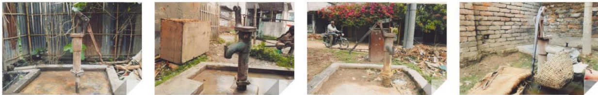
Fig. 27. Hand tubewells fail to extract groundwater because of its sinking down. Or they yield arsenic-contaminated water
