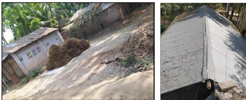
Fig. 13: Corrugated tin shed roofs. Brickbuilt walls have corrugated tin sheds
